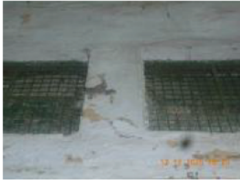
NC_Peeled of plaster at warehouse 1 .jpg
