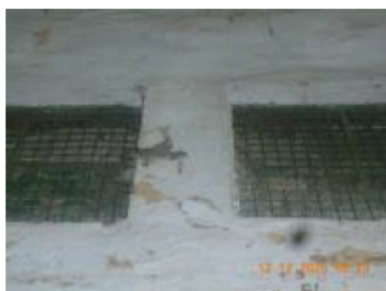
NC_Peeled of plaster at warehouse 1.jpg
