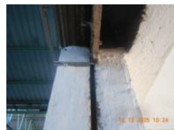
Locking mechanism provided to the Shutter door .jpg
